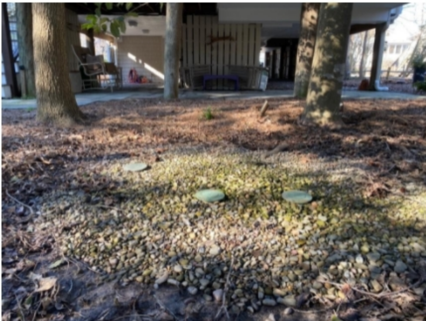
Exterior stone sump away from structures and adjacent to area drainage. Sump pump and gutter drainpipes feed run off water to this one
