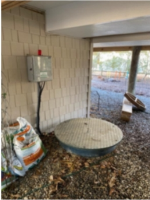
Exterior stone sump away from structures and adjacent to area drainage. Sump pump and gutter drainpipes feed run off water to this one
