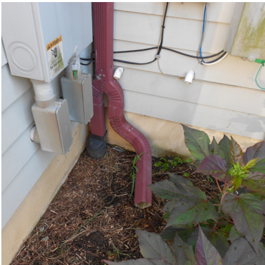
Figure 20: Gutter system to Dry Well This gutter system, installed on a resident's home in Lewes, conveys water to two different locations: a dry well and a rain garden.
