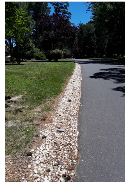
Figure 13: Rolling Road Infiltration Trench
