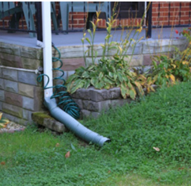
Figure 22: Disconnected Downspout The downspout featured above is an example provided by the University of Maryland Extension.
