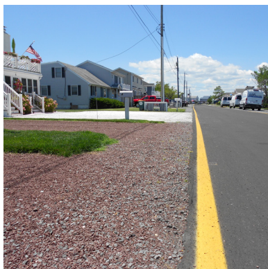
Figure 10: Bayard Street Infiltration Trench The Town of Fenwick Island installed an infiltration trench along Bayard Street to filter and store stormwater before draining to the canal.
