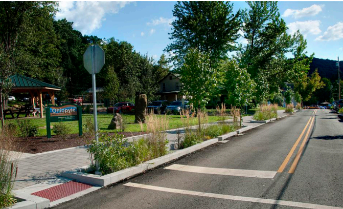
Figure 29: Ohiopyle State Park Trees are planted in a streetscaped bioretention area between the sidewalk and street at Ohiopyle State Park in southwestern Pennsylvania.
