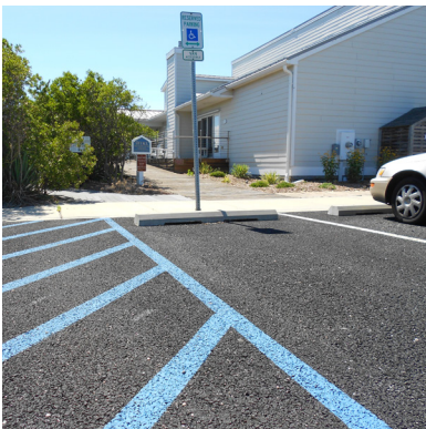
Figure 16: Porous Asphalt at CIB The Delaware CIB's main office is located in a vulnerable location along the Indian River Bay. Their porous asphalt parking lot helps disperse water during high rain events.
