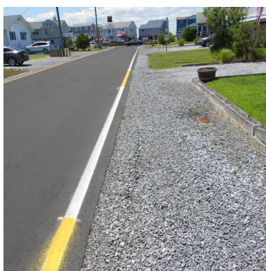
Figure 11: Bayard Street Infiltration Trench Spray paint is used along the street to indicate where parking is and is not allowed even though there is no curb present.
