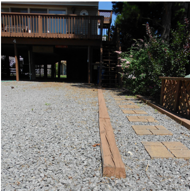
Figure 18: Paver Pathway More and more residents are choosing to use pavers or gravel, which allow infiltration, instead of traditional concrete for driveways and walkways.
